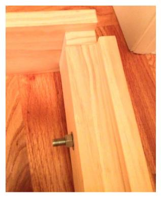
Now you can more clearly see how the ends of the long members look as well. There is a block on the end – it is 1x4 cut to the width of the 2 board sandwich (1 ½ inches). It holds an anchor which the bolts that go through the 1x6 end caps bolt into. That endcap is present on the end of each of the 3 supporting members, so there are 6 endcaps in place. Their construction and attachment is the most labor intensive part of the construction.
